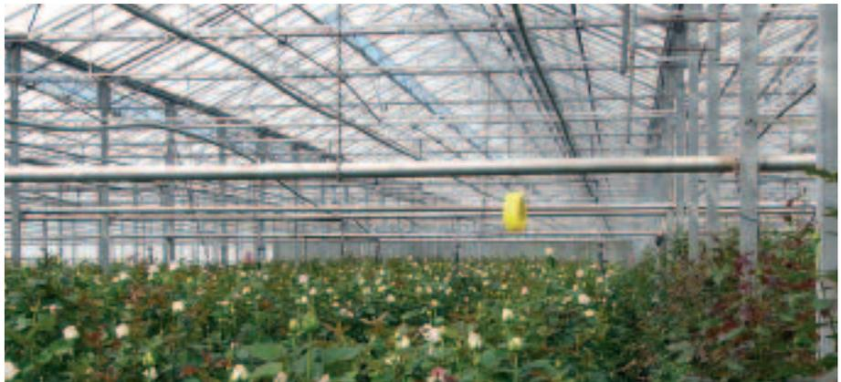
While glass provides better light transmission than most plastic options, its heavier weight requires more substantial structures resulting in shadows that may affect the crop.
